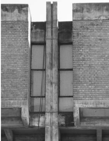
▲ 10.18 Full-height windows adjacent to columns suggest another means of creating vertical gaps between infill walls and columns. Library building, Kanpur, India.
