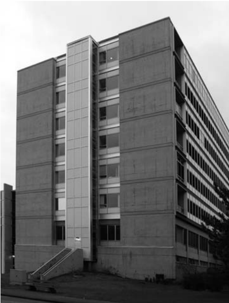
▲ 12.13 External retrofitted concrete shear walls, Vancouver.
