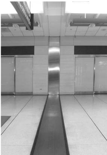
▲ 8.28 A seismic joint between floors, walls and ceilings of two separated structures, San Francisco.
