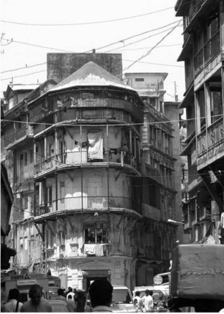
▲ 16.2 Seismically vulnerable buildings in Mumbai. (Reproduced with permission from R. Sinha).
