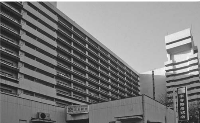
▲ 15.6 Two of an irregular line of eighteen apartment blocks forming a firewall protect a refuge area. During a fire, metal shutters cooled by falling water protect the glazing. Shirahige, Tokyo. (Reproduced with permission from Geoff Thomas).
