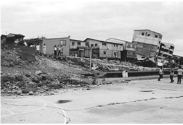
▲ 1.5 A surface fault with considerable vertical displacement. The 1999 Chi Chi, Taiwan earthquake. (Reproduced with permission from Chris Graham).
