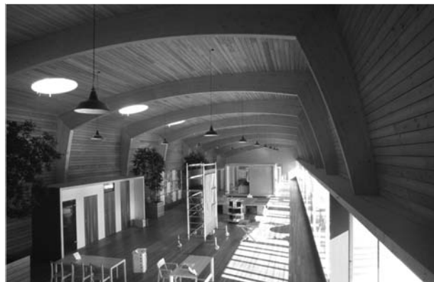
▲ 5.41 An elegant wood moment frame. Commercial building, Austria.
