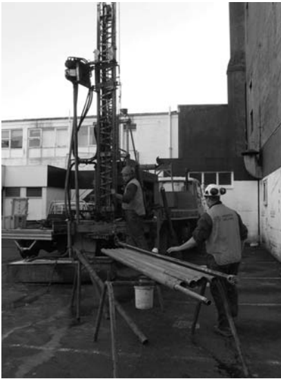
▲ 7.9 A drilling crew undertaking foundation investigations. Wellington, New Zealand.
