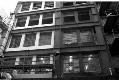
▲ 12.16 An external steel moment frame retrofit, Wellington.
