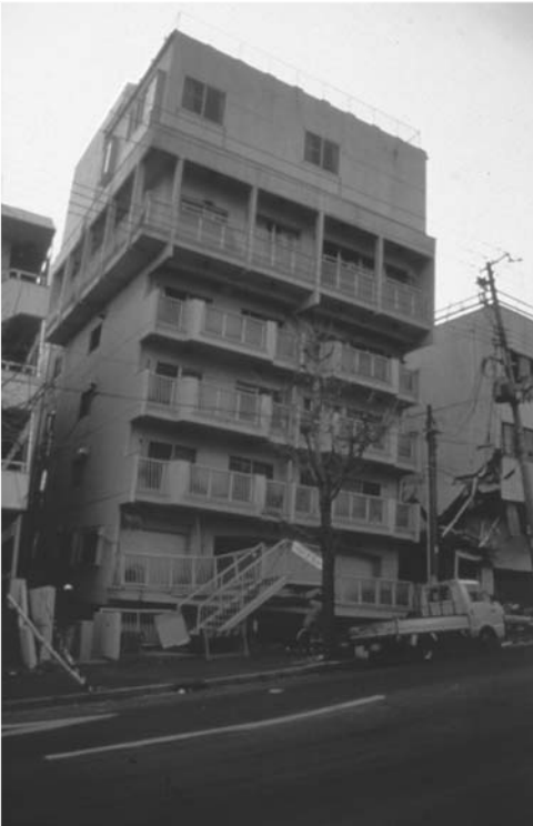
▲ 8.1 Collapse of a concrete frame building at ground floor level due to torsion, 1995 Kobe, Japan earthquake. (Reproduced with permission from EERI, David R. Bonneville, photographer).
