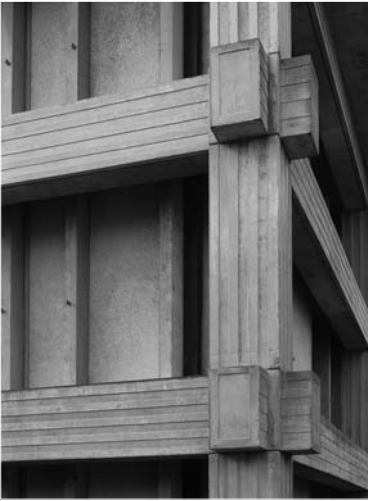
▲ 17.5 Typical beam studs. Educational building, Wellington.
