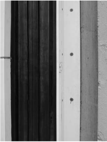
▲ 8.25 Concertina flashing between two buildings, San Francisco.
