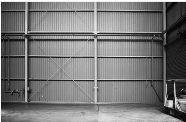
▲ 5.24 Tension-only bracing. Light industrial building, Wellington.
