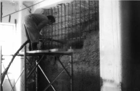
▲ 12.11 Shotcreting to form a new internal reinforced concrete wall, Wellington.
