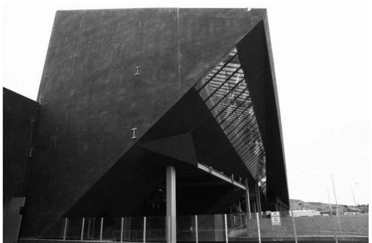
▲ 6.19 The Stealth Building whose cross-sectional form morphs from triangular to square along its length. Los Angeles.
