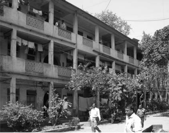
▲ 16.5 Slender columns can not provide adequate seismic resistance. Mumbai. (Reproduced with permission from R. Sinha).
