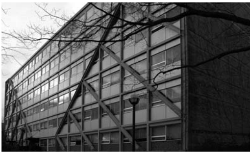
▲ 12.14 External retrofitted braced frames, Vancouver.
