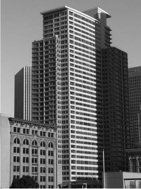
▲ 14.23 Post-tensioned unbonded tendons provide a damage avoidance mechanism in most of the moment frames of this 39-storey apartment and retail building, San Francisco.
