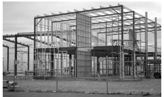
▲ 5.15 A two-storey wood shear wall with steel chords. Wanganui, New Zealand.
