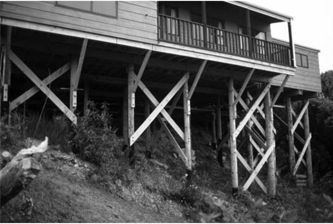
▲ 5.28 Sub-floor wood bracing of a wood framed house. Wellington.
