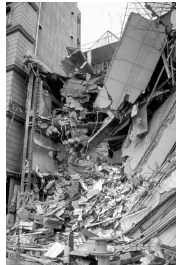
▲ 3.3 Brittle structural damage, Kobe. 1996 Kobe, Japan earthquake. (Reproduced with permission from Adam Crewe).
