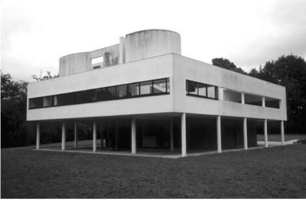
▲ 3.6 Villa Savoye, Poissy, Paris, Le Corbusier, 1929. This villa incorporates all of Le Corbusier's 'five points' of architecture. A combination of pilotis and irregularly placed concrete block walls resist horizontal forces.
