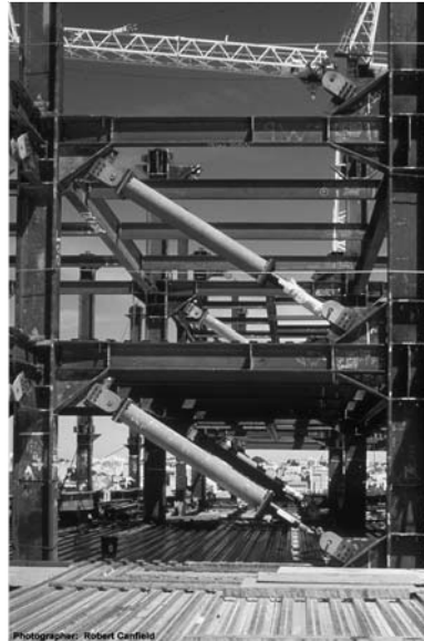
▲ 14.17 Dampers placed at the ends of tubular steel braces. Office building, San Francisco. (Reproduced with permission from David Friedman, R. Cranfield, photographer).
