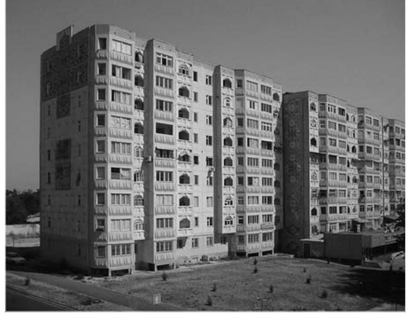
▲ 16.3 Frame and panel buildings in Tashkent that may not meet current seismic standards. (Reproduced with permission from Nadira Mavlyanova).
