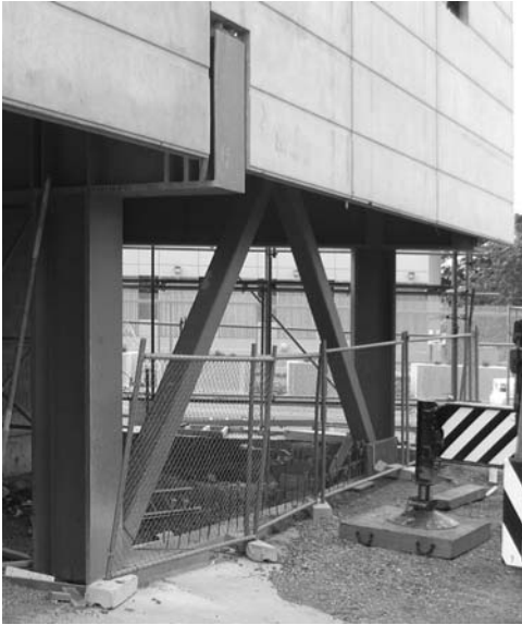
▲ 4.16 A hidden eccentrically braced frame immediately behind precast concrete panels is offset from the ground floor braced frame. A short transfer diaphragm moves horizontal shear from the outer frame to the inner ground floor frame (Left). To resist the overturning-induced compressions and tensions from columns above, the first floor cantilever beams are very deep (Right). Apartment building, Wellington.
