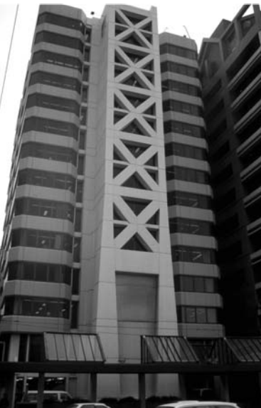
▲ 5.29 Reinforced concrete tension and compression bracing. A high level of collaboration between the architect and structural engineer achieved the gradually reducing brace dimensions up the height of the structure. Office building, Wellington.
