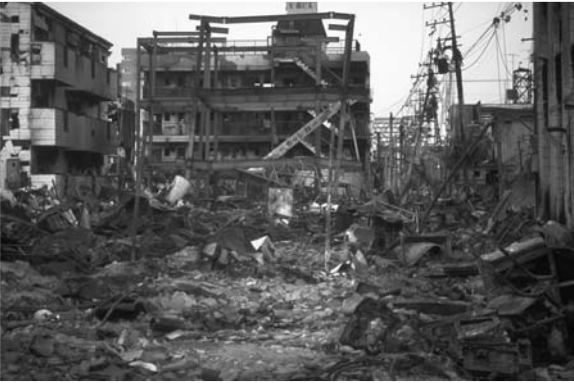
▲ 15.5 A localized example of fire damage following the 1995 Kobe, Japan earthquake. (Reproduced with permission from Adam Crewe).
