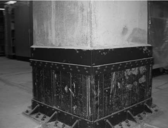
▲ 14.14 A lead-rubber bearing inserted at the base of a reinforced concrete column.
