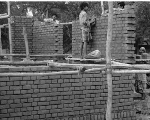
▲ 5.14 An unreinforced masonry wall under construction. Kanpur, India.
