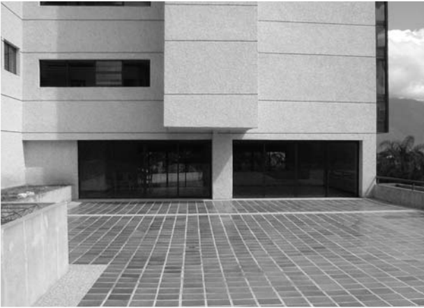
▲ 16.4 Soft storey building, Venezuela. (Reproduced with permission from Wiss, Janney, Elstner Associates, Inc.).
