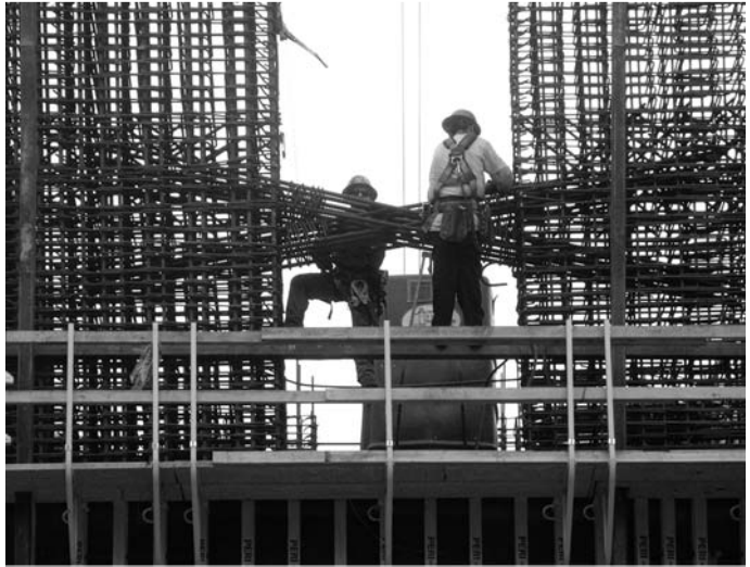
▲ 5.22 Diagonal reinforcement in a coupling beam. Office building, San Francisco.
