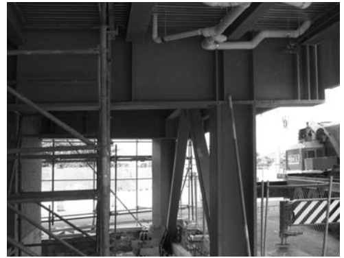
▲ 4.16 A hidden eccentrically braced frame immediately behind precast concrete panels is offset from the ground floor braced frame. A short transfer diaphragm moves horizontal shear from the outer frame to the inner ground floor frame (Left). To resist the overturning-induced compressions and tensions from columns above, the first floor cantilever beams are very deep (Right). Apartment building, Wellington.
