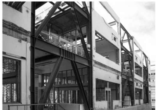
▲ 12.15 Eccentrically braced frames strengthen a reinforced concrete building, Wellington.
