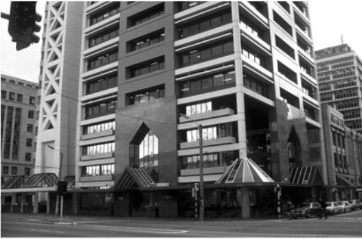
▲ 6.8 Seismic forces are resisted by two one-bay moment frames in each orthogonal direction. Shallow beams and slender columns support gravity forces. Office building, Wellington.
