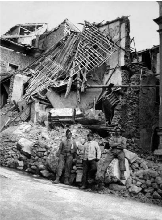
▲ 3.1 Damage to the city of Messina from the 1908 earthquake. (Reproduced with permission from Arturo Tocchetti; copyright Russell Kightley).
