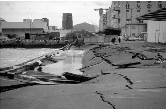
▲ 7.5 Lateral spreading damage to harbour pavements. 1995 Kobe, Japan earthquake. (Reproduced with permission from Adam Crewe).
