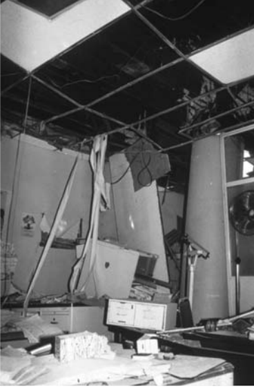
▲ 11.26 Damaged office contents. Mexico City, 1985 Mexico earthquake (Reproduced with permission from David C. Hopkins).
